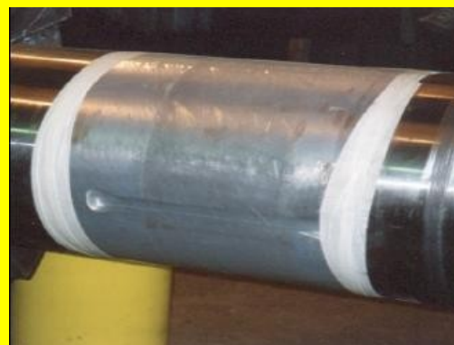
Sealing holes in pipe
