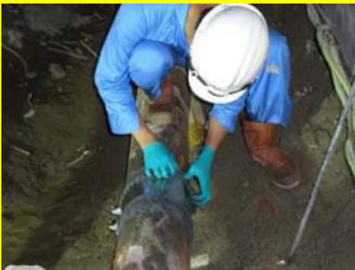
Filling up gaps
