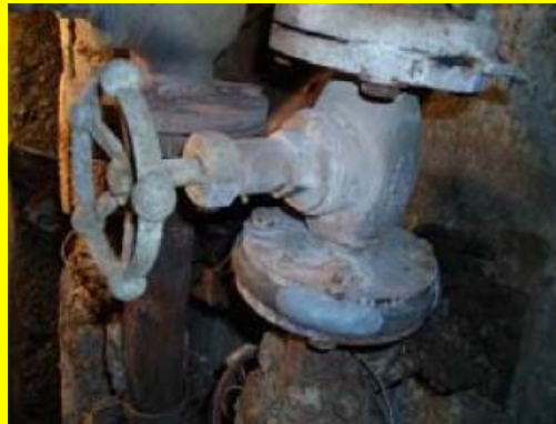
Sealing pipe flanges
