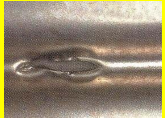
Filling cracks on surface
