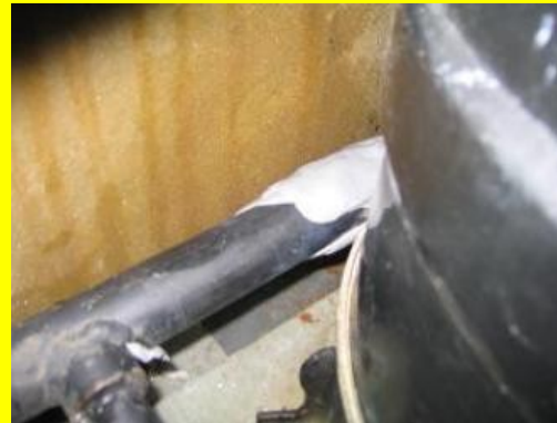
Sealing holes in pipe
