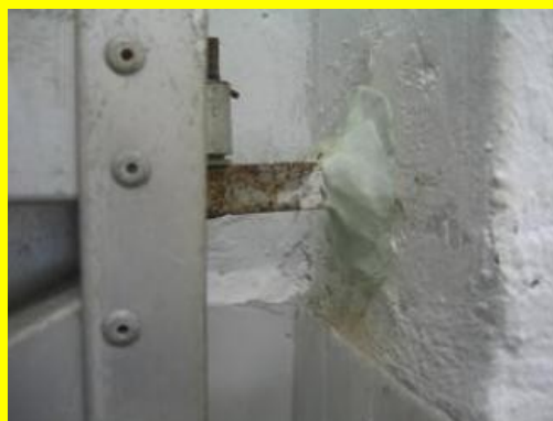
Filling up holes in wall
