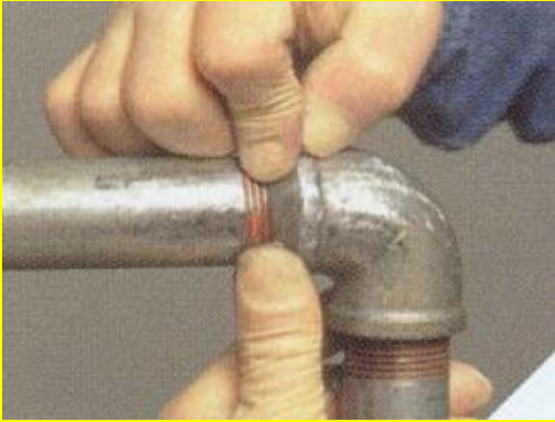
Filling up pipe threading
