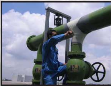
Tee-Joint Repair
