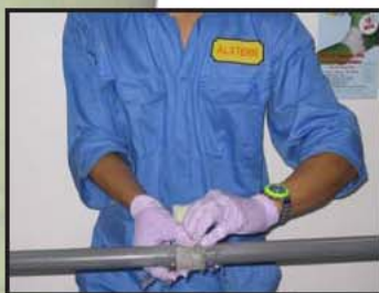
• Wrapping the leak area with WRAP SEAL™
