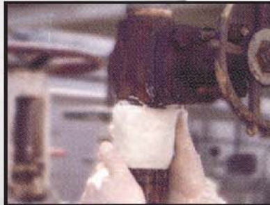
Valve Thread Repair
