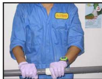
• Polishing the repaired area
