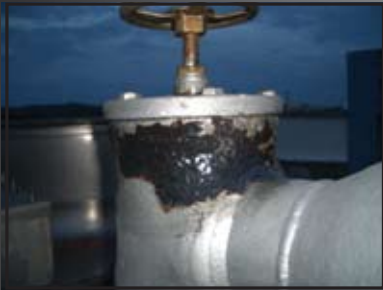
Tee-Joint Repair
